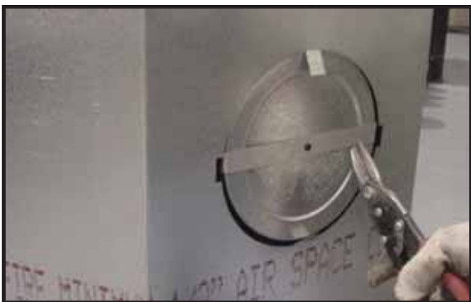
Figure 9.9 Cut the metal retaining band and fold the sides out.
